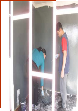
Painting the walls at Pat-son’s new home at Crossroads
